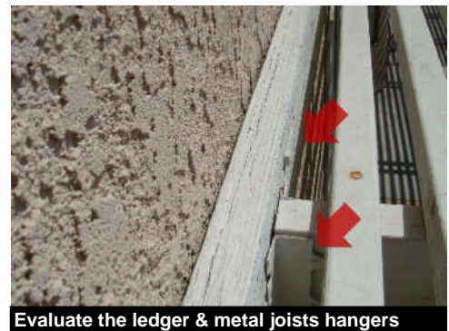
Evaluate the ledger & metal joists hangers
