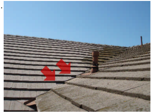
Broken rake tile. Evaluate water stains.
