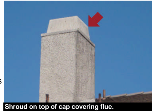
Shroud on top of cap covering flue.
