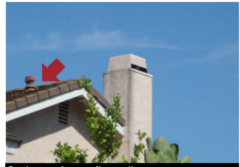
Seal water heater flue collar.
