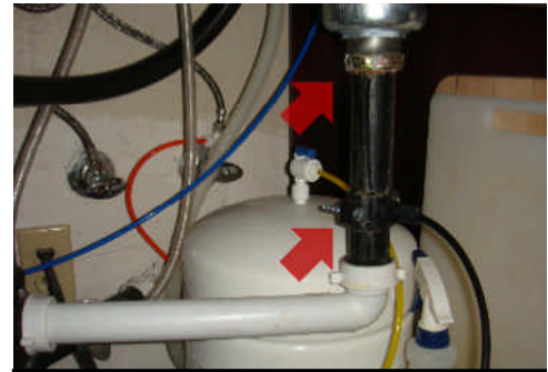
Improper saddle clamp on drain pipe.
