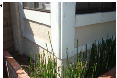
Soil above the interior slab /flooring.
