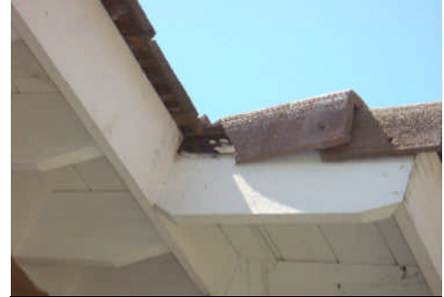
Broken rake tile. Evaluate water stains.
