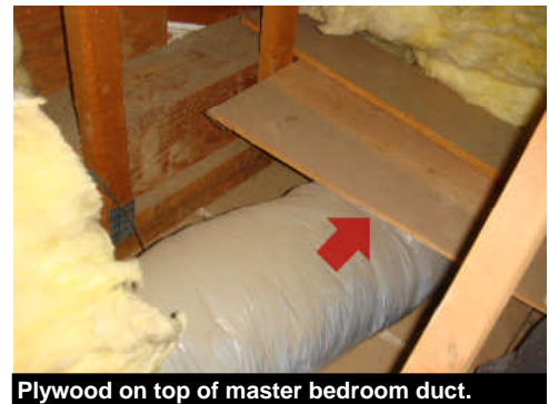
Plywood on top of master bedroom duct.
