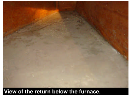
View of the return below the furnace.
